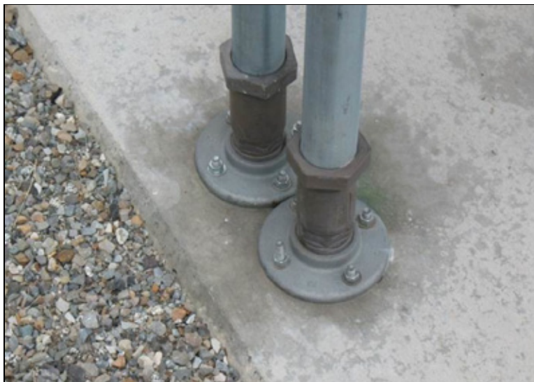
Figure 6-2. Two frangible connections
